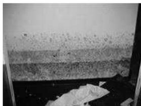
**Mold on wall extends above flood level because the moisture wicked up the drywall.**
