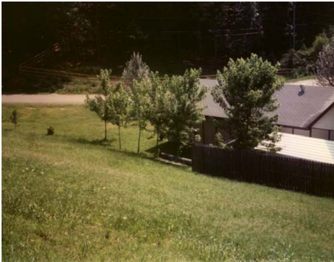
FIGURE 3.1 House immediately below earthen dam
