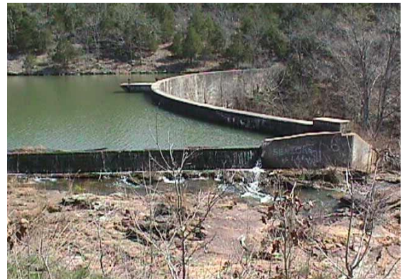
b. Concrete arch dam
