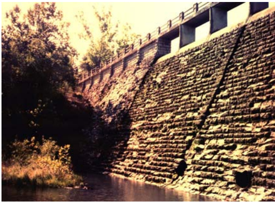
a. Rock-filled gravity dam
