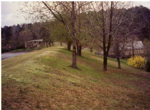
c. Small earthen dam
