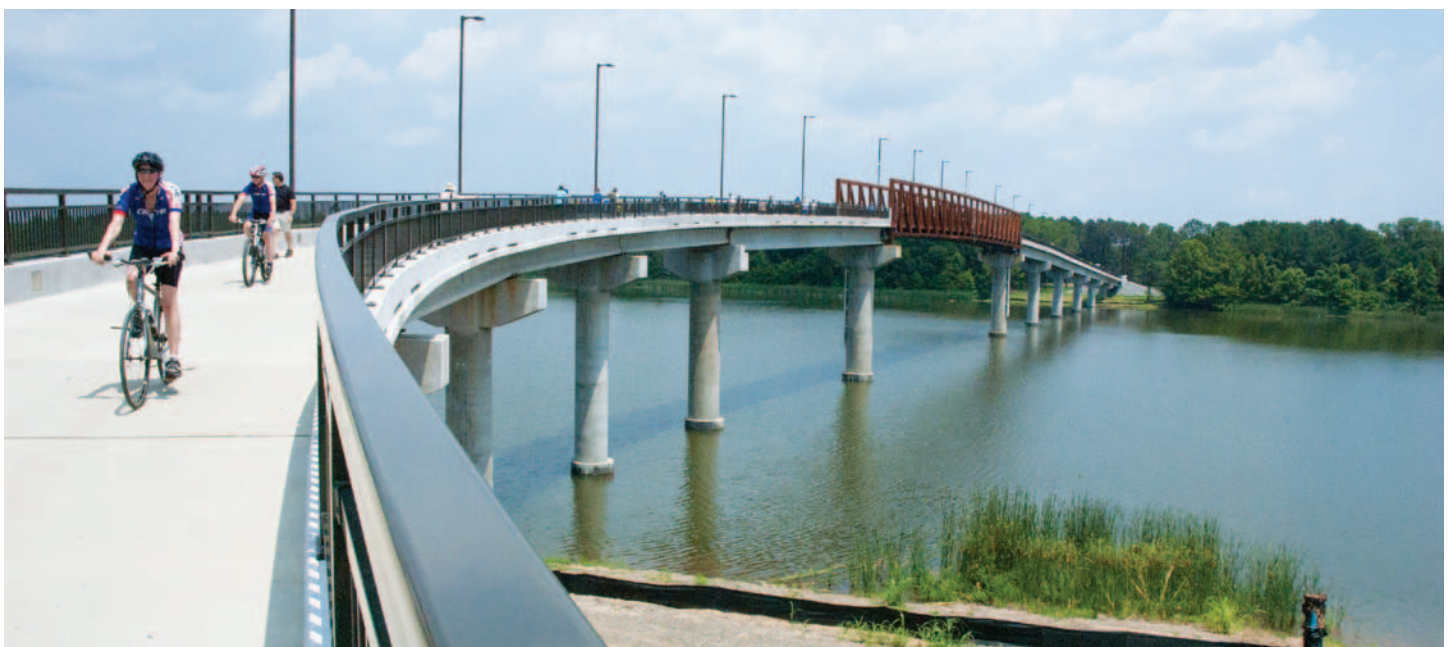
Dozens of cyclists, runners and walkers turned out July 8 to be among the first to cross the new Two Rivers Bridge, which opened to the public July 23.
