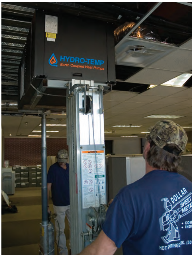
Bryan Lillard, left, and Jackie Hill, of Benton-based Jones Heating and Air, install a geothermal heat pump into the ceiling at League headquarters in North Little Rock.
