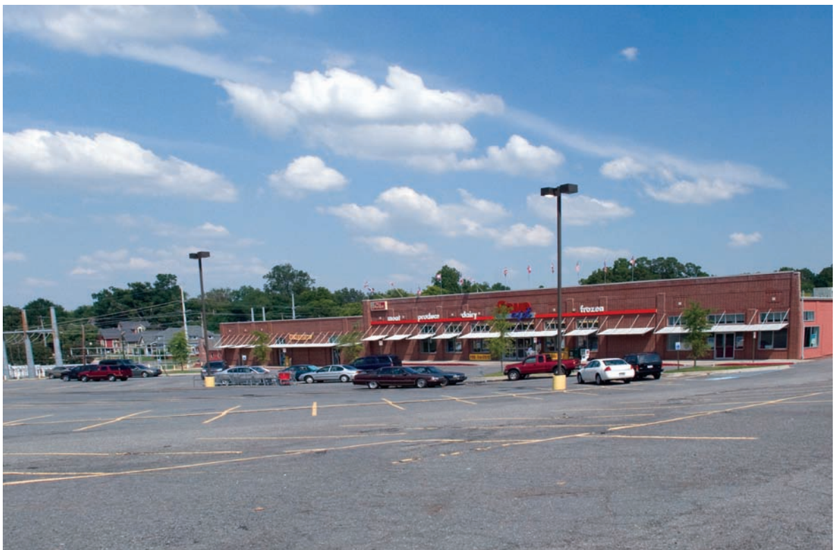
This parking lot at the corner of Broadway and Roosevelt Road in Little Rock is far too big for the business it serves. Not only is the space wasted, it makes the city hotter and the unused asphalt pours pollutants into our streams and rivers.
