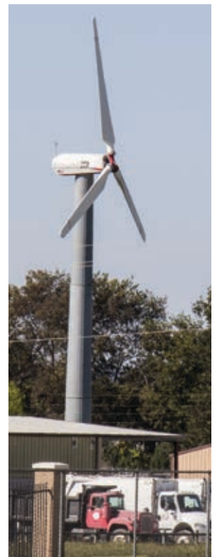
Arkansas Wind and Solar's windmill is a landmark at the city's thriving industrial park.
