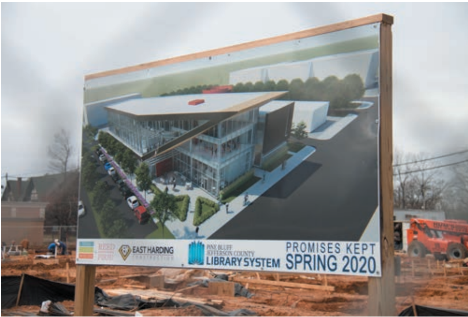
Construction has begun on Pine Bluff's new main library, which city leaders believe will help continue downtown's rebirth.
