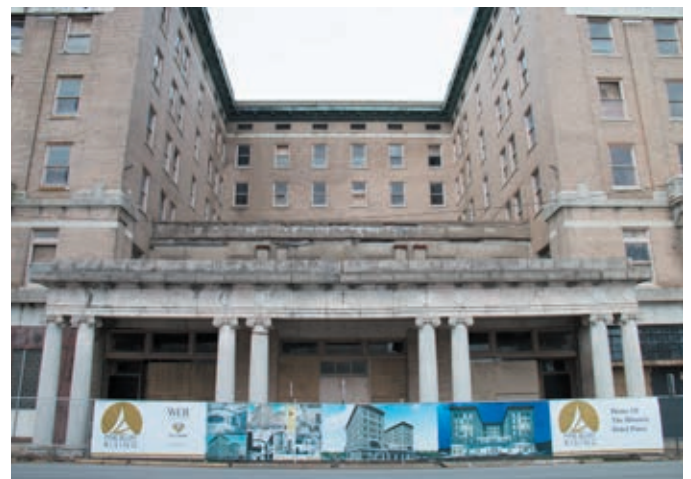
Renovation of the historic Hotel Pines is another piece of the revitalization efforts.
