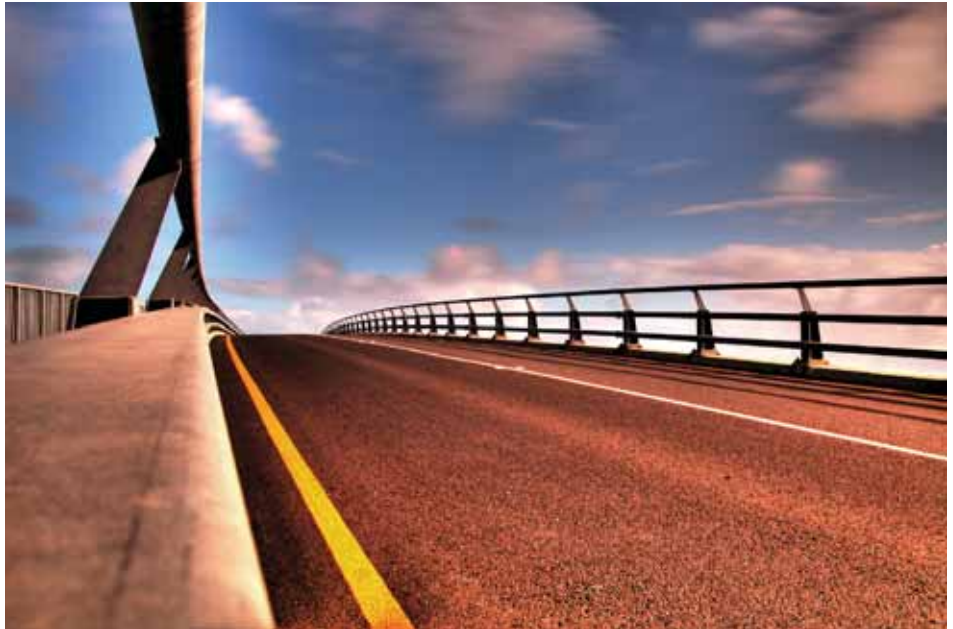
Coatings on bridges can help protect against chemical reactions.
