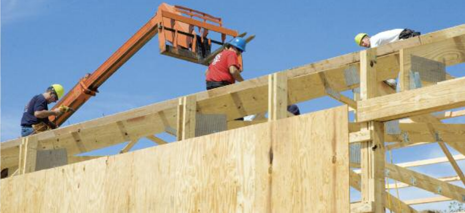
Workers frame the roof of Mena's new 4-H community center.
