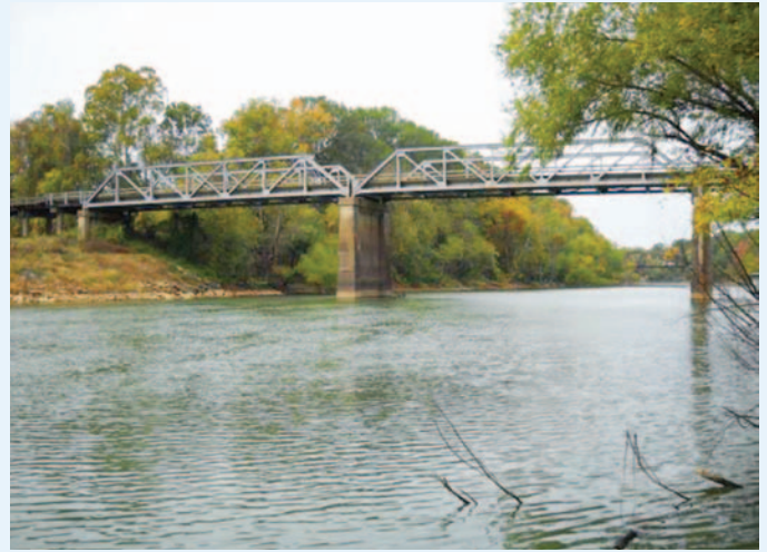
To extend water to new customers at Harmony Grove, Camden is boring underneath the Ouachita River.
