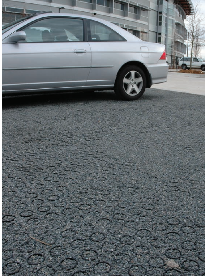
Even Heifer’s parking lot is environmentally friendly—porous to minimize runoff and allow underground capture of the water for other uses.
