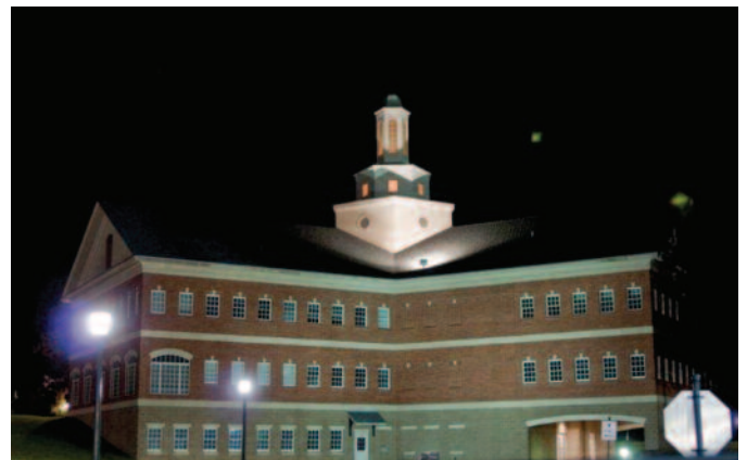
The Arkansas State University - Mountain Home campus is experiencing unprecedented growth at this time.
